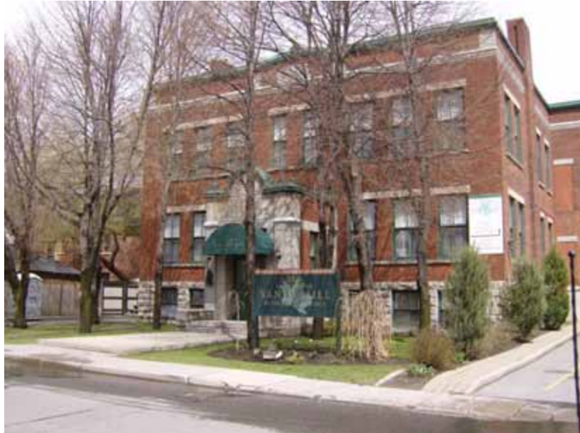
34 Former École St.-Pierre, 353 Friel Street, now La Résidence Sandy Hill Retirement Residence; built in 1906, closed as a school in 1930. (Bruce Macdonald, 29 April 2007.)
