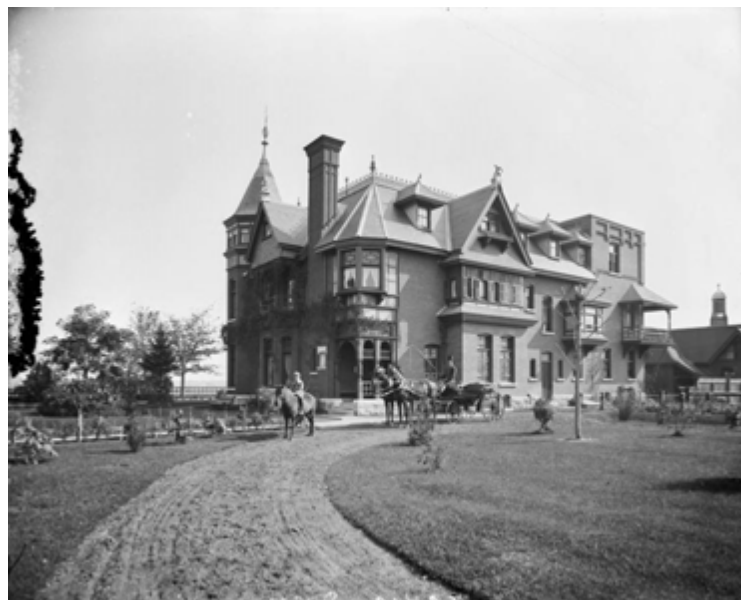
25 The W. H. Davies residence, 404 Theodore/Laurier Avenue East at the corner of Marlborough, ca. 1895, was among the first of the grand residences in the former By estate. (NLA, PA27700.)
