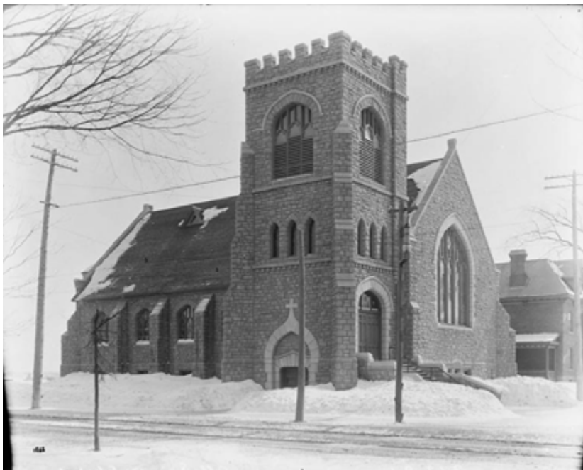
32 All Saints Anglican Church, 315-317 Chapel Street at Laurier Avenue East; built in 1899-1900, A. M. Calderone, architect, ca. 1900. (NLA, PA09034.)
