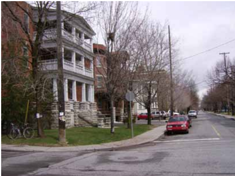
38 The three apartment buildings at 253-255-257 Daly Avenue illustrate the design of early multiple-family buildings within the SHHS. (Bruce Macdonald, 29 April 2007.)
