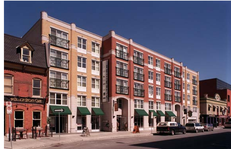
Figure 13: An Ottawa example of a 5-storey building designed to reflect a variety of buildings while avoiding the monolithic look of one long block.
