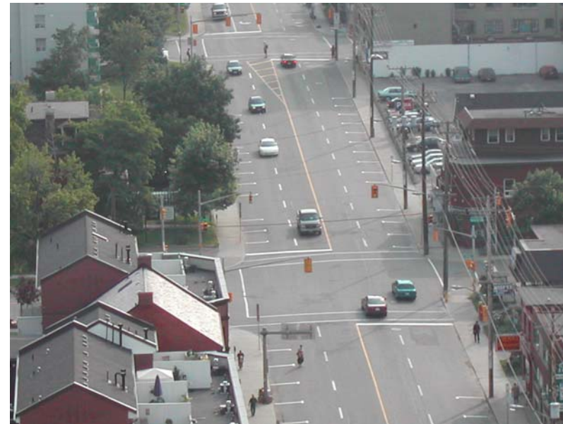
Figure 4: Existing conditions on Rideau Street at Cobourg Street.
