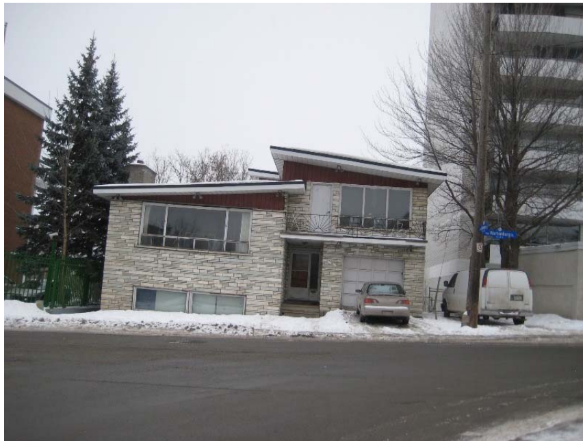
Photograph 1: View looking east, facing Wurtemberg Street towards the front of the Site (101 Wurtemberg Street).
