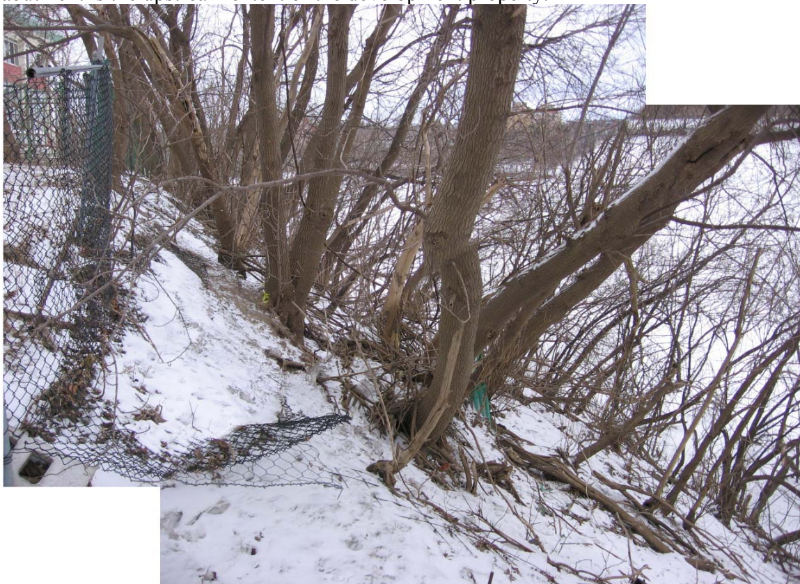
Photo 2. View across the slope on February 21, 2010. The fence represents the top of the slope on the development property.
