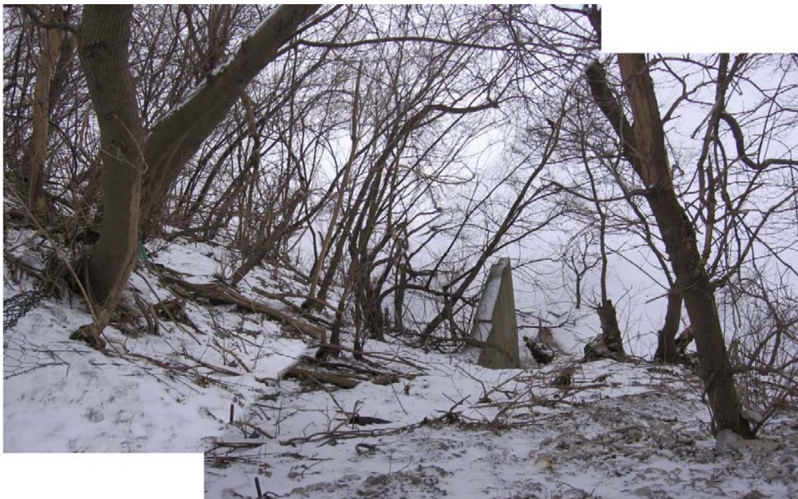
Photo 1. View down slope to the Rideau River on February 21, 2010. The concrete abutment is the upstream extent of the development property.
