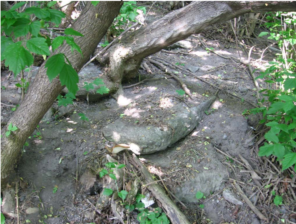
Photo 17. Eroding slope above the shoreline – May 25, 2010.
