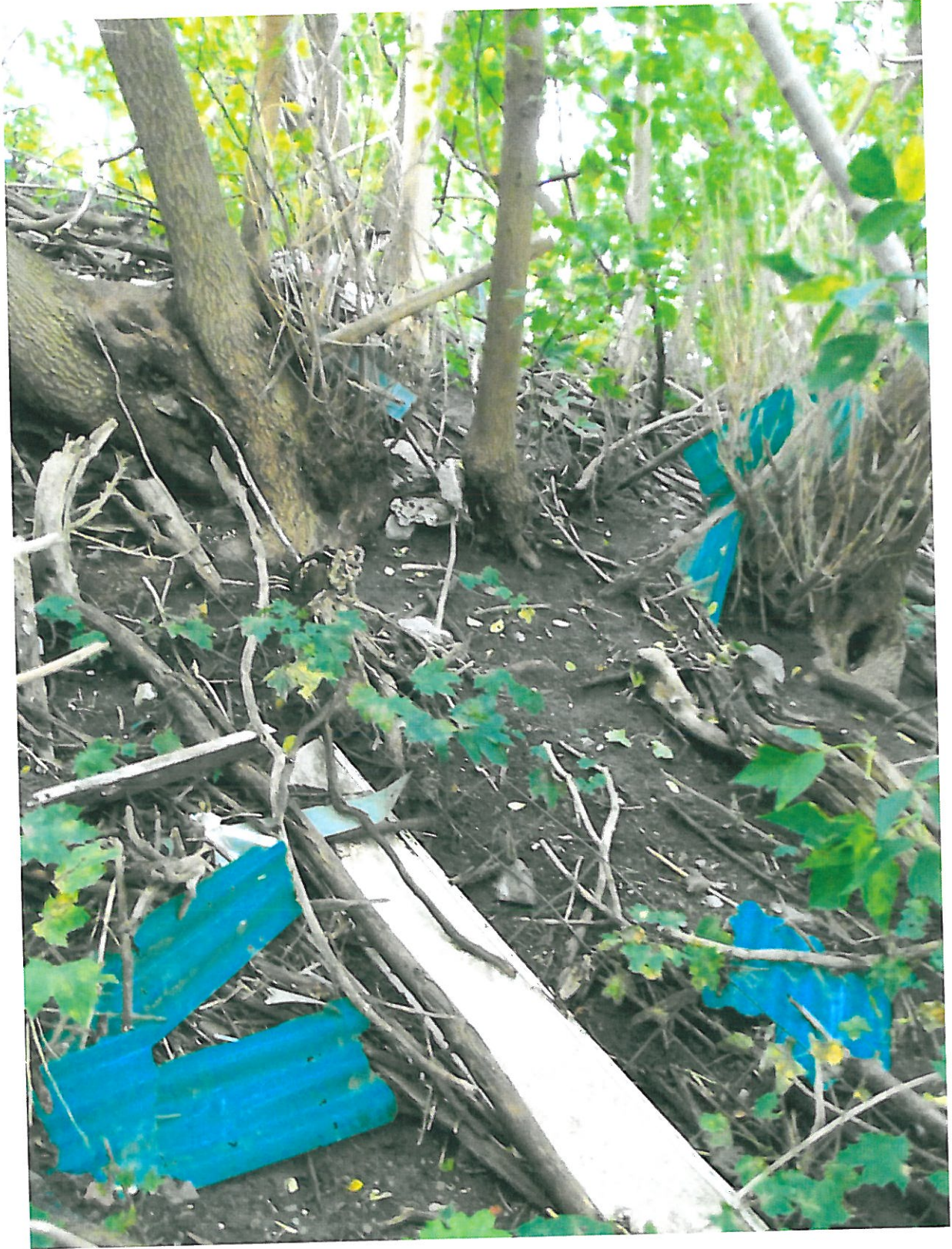
Photo 3. Close-up of slope near the crest
