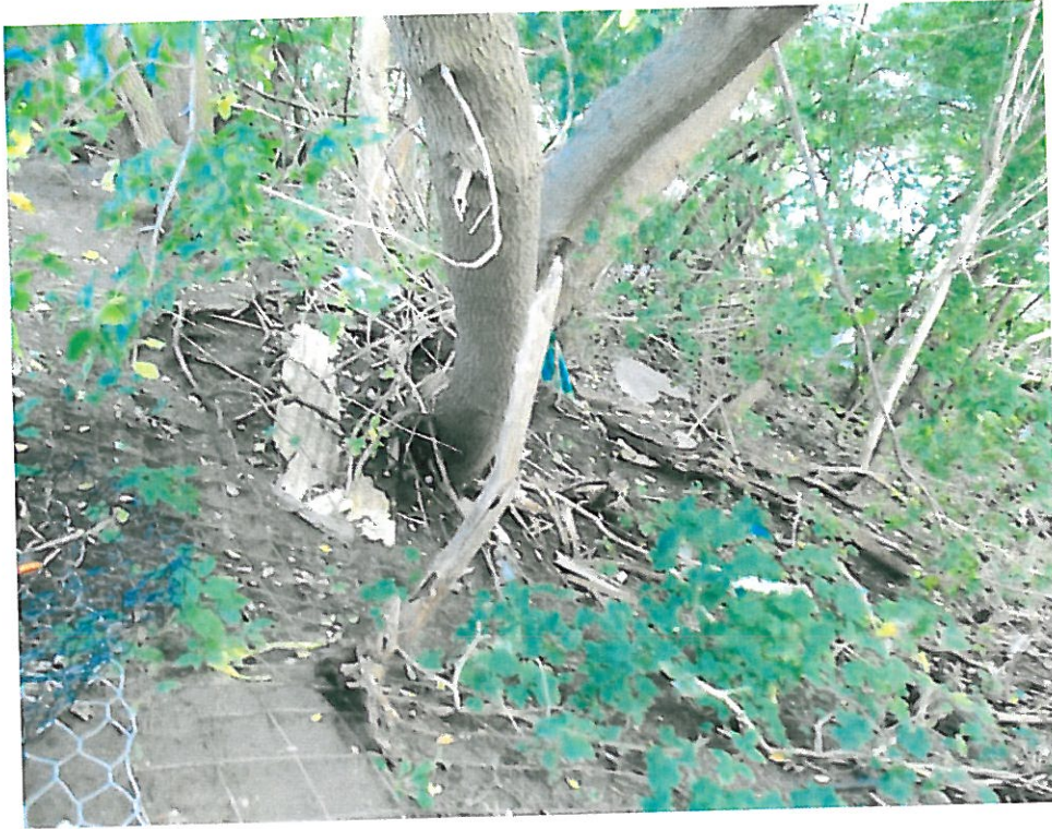
Photo 4. View of crest of slope looking north.
