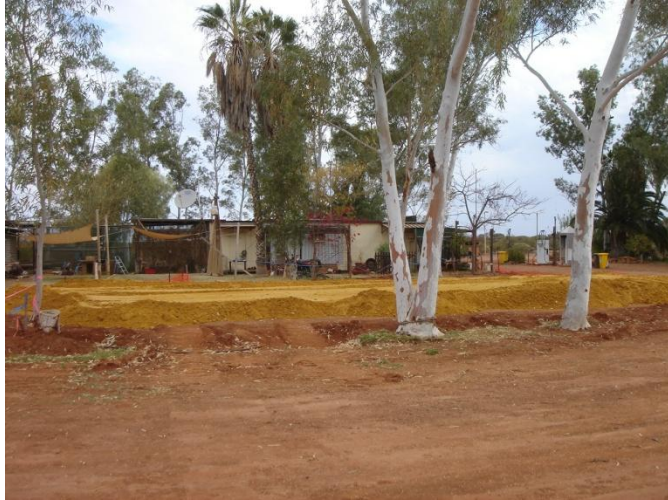
The sand pad for the new roadhouse.
