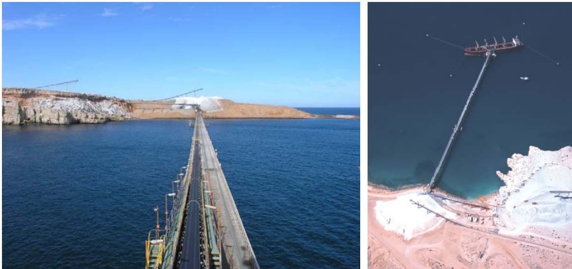
Ship to Shore and Aerial View Photos of the Lake MacLeod Ship Loading Facility.
