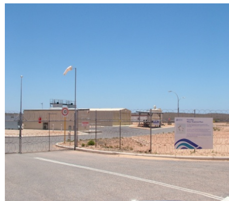
Coral Bay Water Treatment Plant
