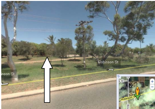
Dual use Pathway in background. This pathway has no effective lighting for most of its entire length along Robinson St.
