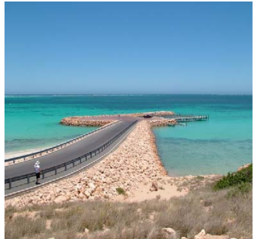
Coral Bay Boat Launching Facility
