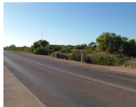
Reid Street Floodway
