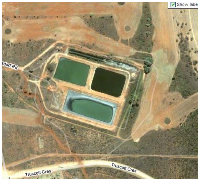
Exmouth Waste Water Treatment Plant. The Golf Course Bounds the North and East
