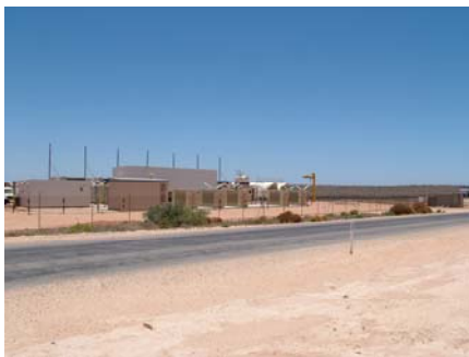
Coral Bay Power Station
