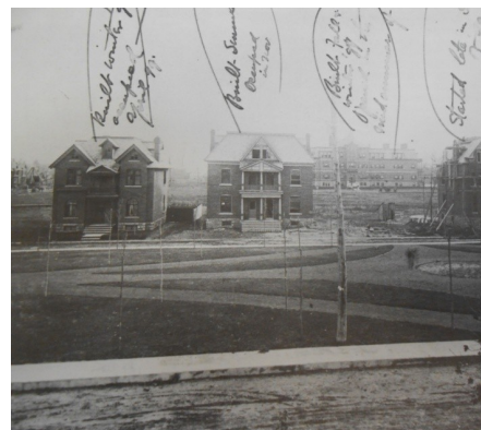
(Minto Park Houses Under Construction late 1800's)
