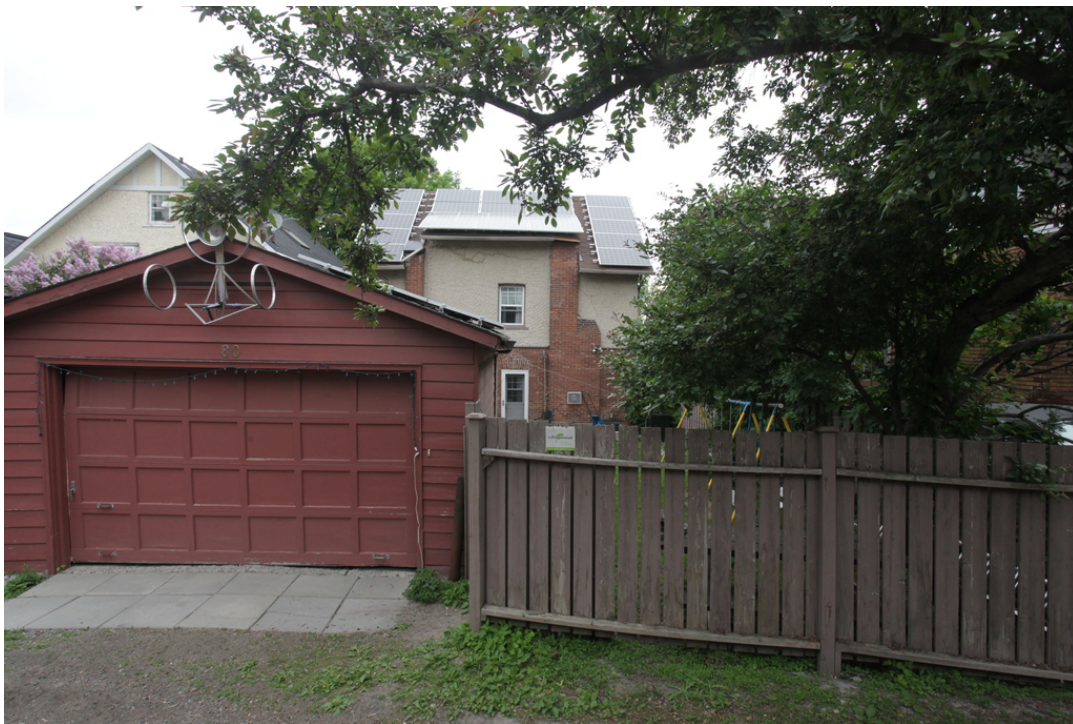
The 1975 garage showing the solar panels on the roof of the house. The original metal siding on the garage has been replaced with clapboard.
