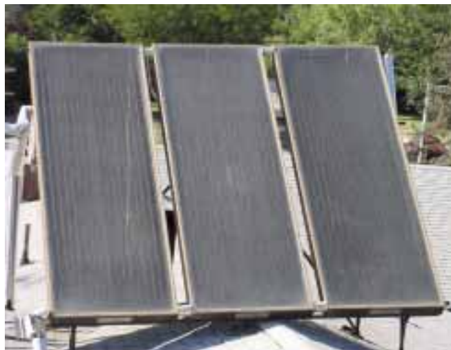
Three, 3 by 8 foot collectors and piping, draining to the left.
