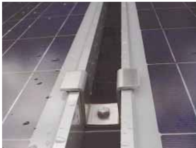
Custom U-brackets hold down adjacent panels.
