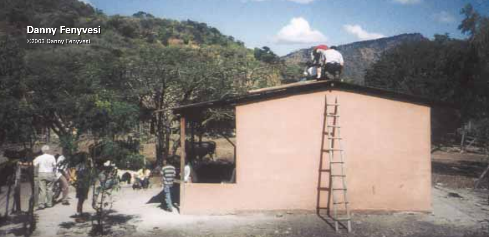
Grupo Fenix workshop participants install a 50 watt photovoltaic panel for lighting on the health clinic in the little village of Las Pintadas, Nicaragua.
