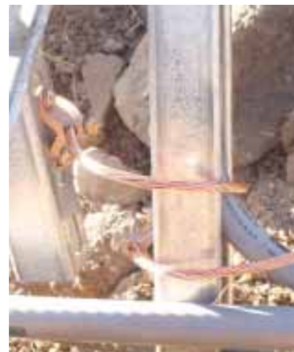
The grounding technique for attaching copper wire to steel in concrete.
