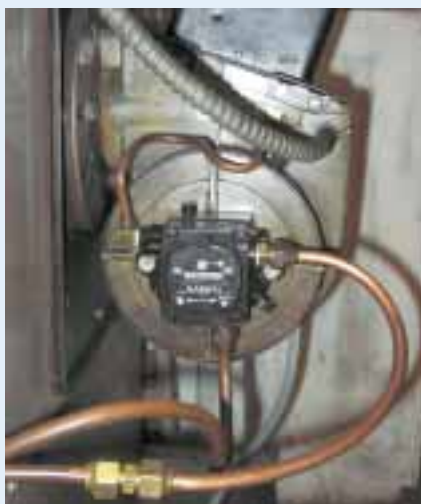
The 30-year-old furnace's new pump has Viton seals to accommodate biodiesel.
