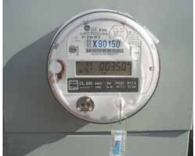
The time-of-use meter shows that when Vincent took the photo he was selling at the rate of 3.5 KW to PG&E.
