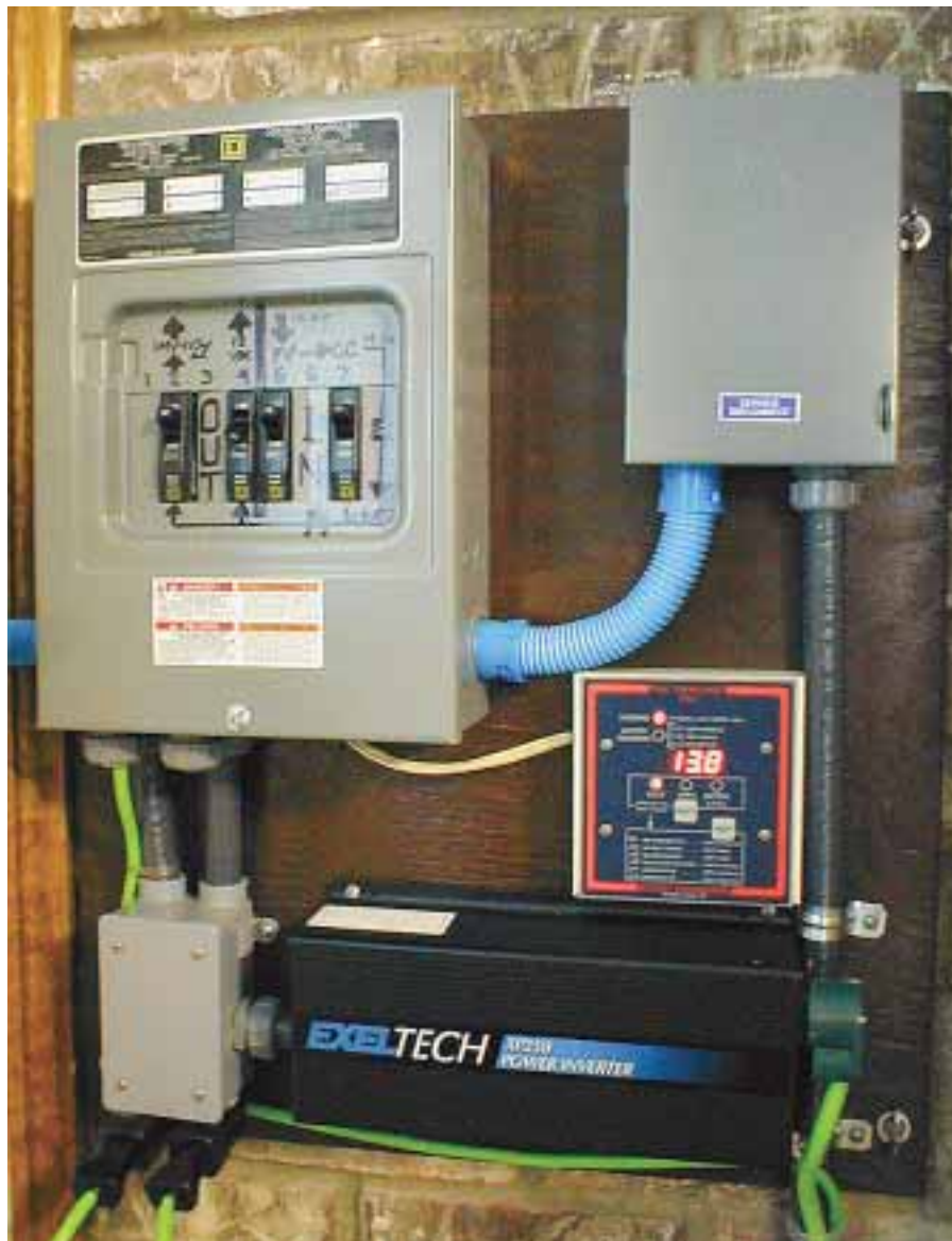
System electrical panel with breaker box, main fused disconnect box, TriMetric meter, Exeltech inverter, and two, DC output jacks.
