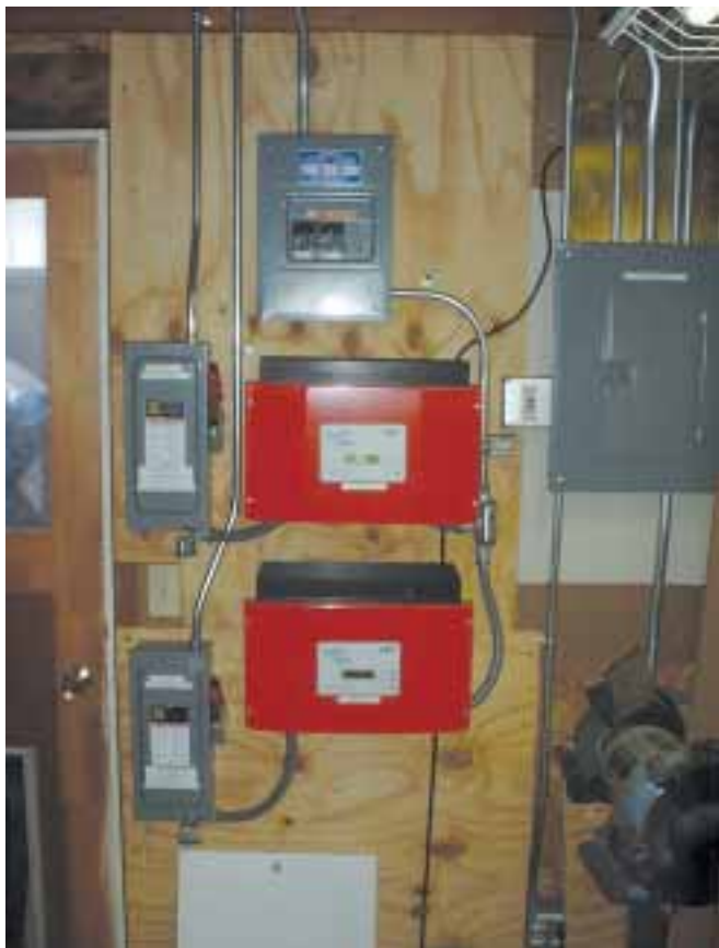
Two SMA Sunny Boy 2500 inverters, two DC disconnects, and the AC panel.
