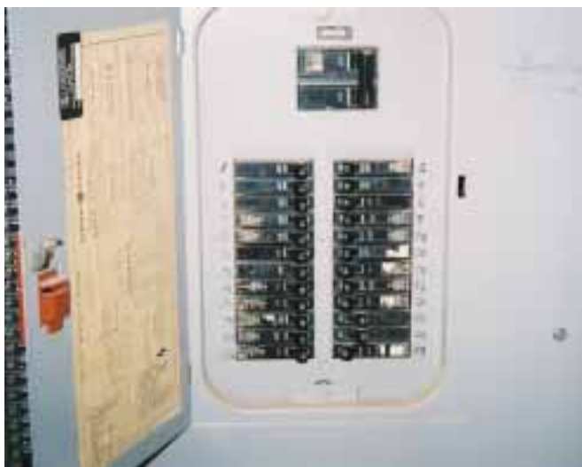
A load center with an AC service disconnect.
