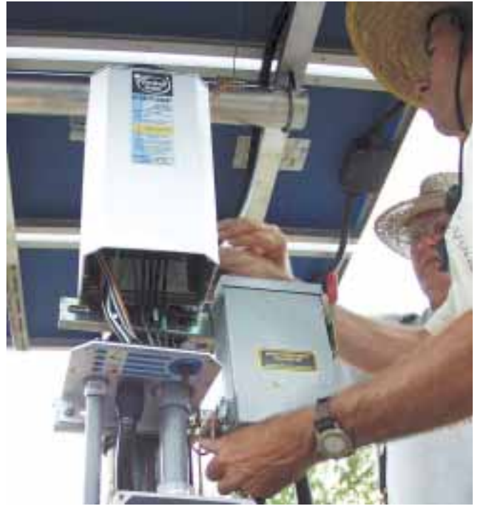
The pump controller wired.
