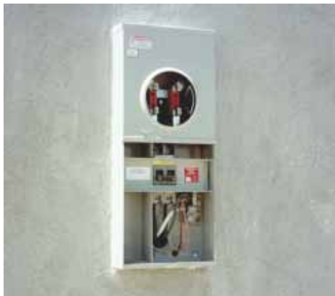
An AC service disconnect, with the meter yet to be installed.
