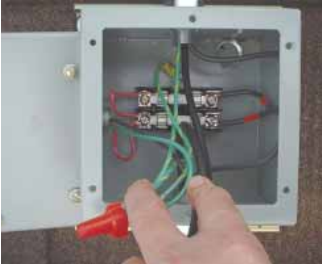
One of the homemade combiner boxes with 10 A, DC-rated fuses.
