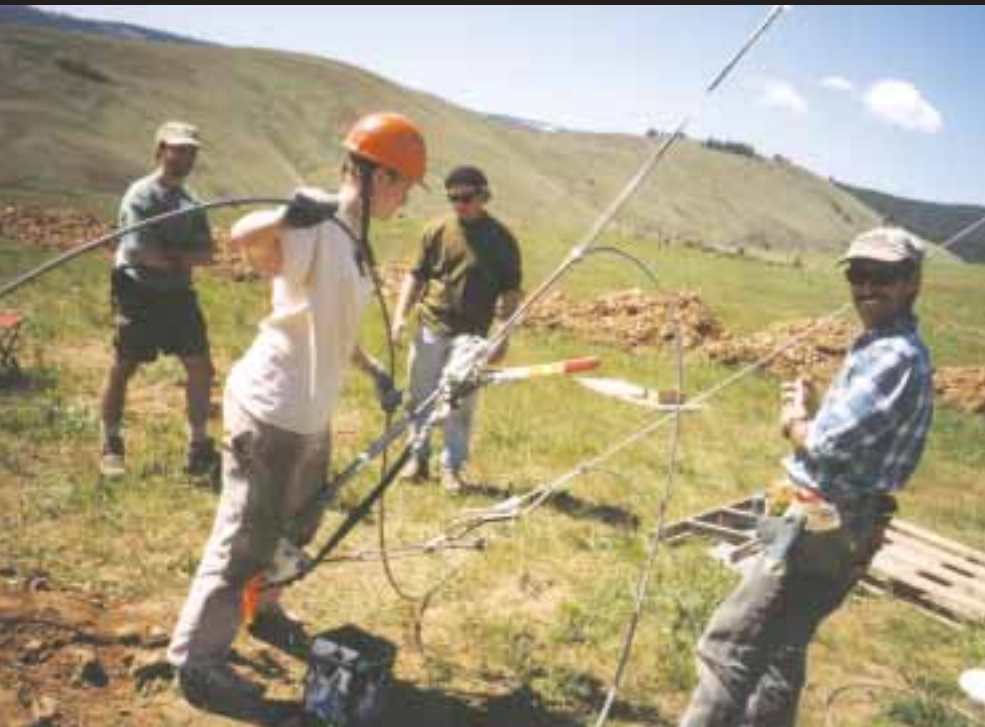
Tensioning the guy wires and plumbing the tower.
