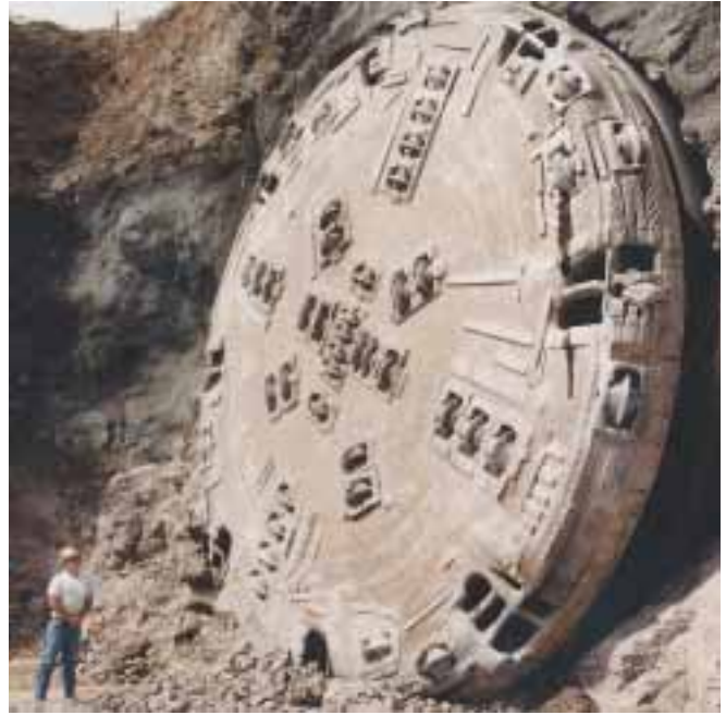
The business end of the boring machine breaks out of solid rock at the South Portal.
