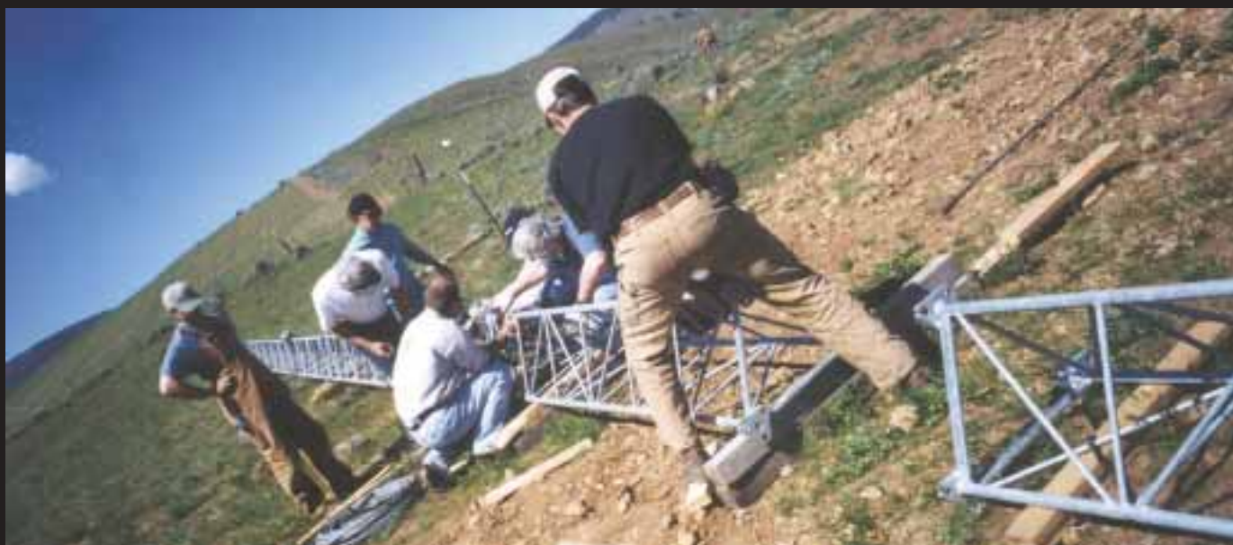
Laying out and bolting together the ten, 10 foot tower sections.
