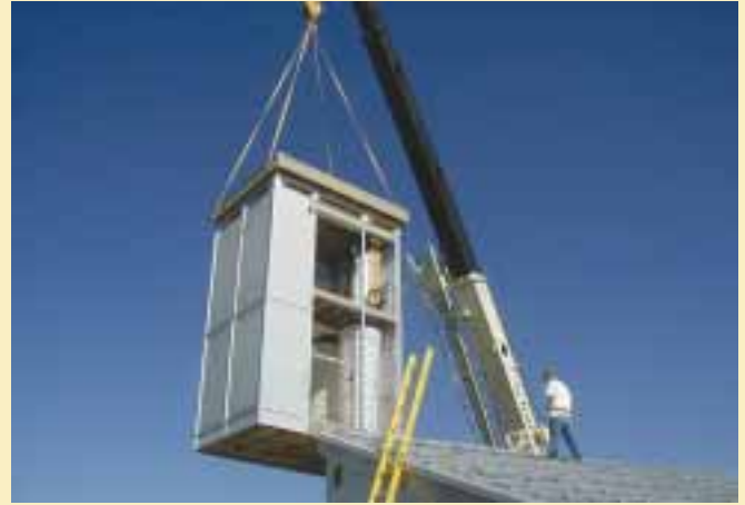
Colorado's tech pod being hoisted in place. You can see the water storage tanks and hot water tank in the upper section.
