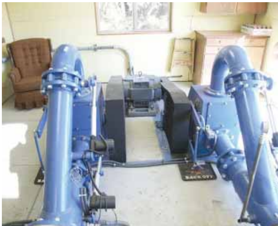
The two Canyon Industries turbines flank the 30 KW, three-phase generator.
