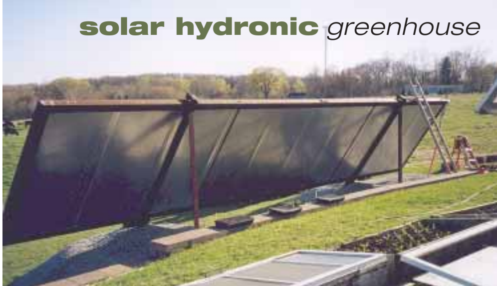
The 8 by 40 foot maxi-collector is all one unit, custom built for the greenhouse.
