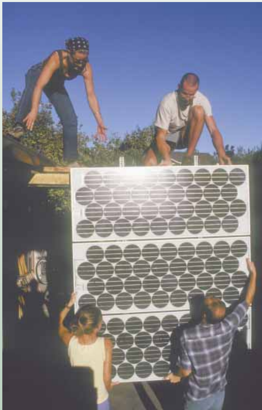
The de-installation crew lowers the rack and PVs—Tiffany, Scott, Nicole, and Scott. We designed the system to be easily movable because when you move a lot, what goes up, must come down.
