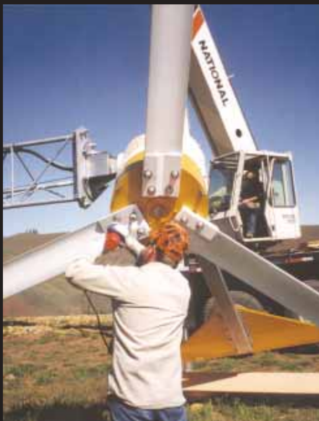
Mounting the blades using an impact wrench.
