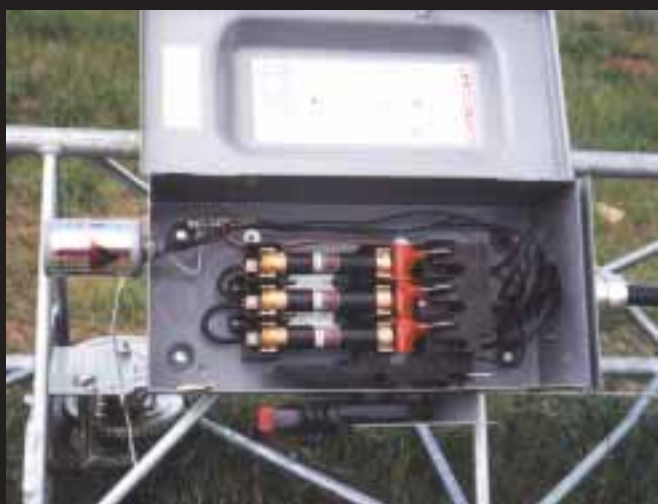
Overcurrent protection at the tower's base.
