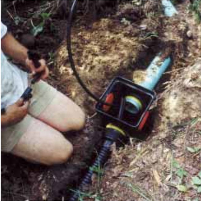
Clean-out boxes help with distribution of irrigation water, as well as system maintenance.
