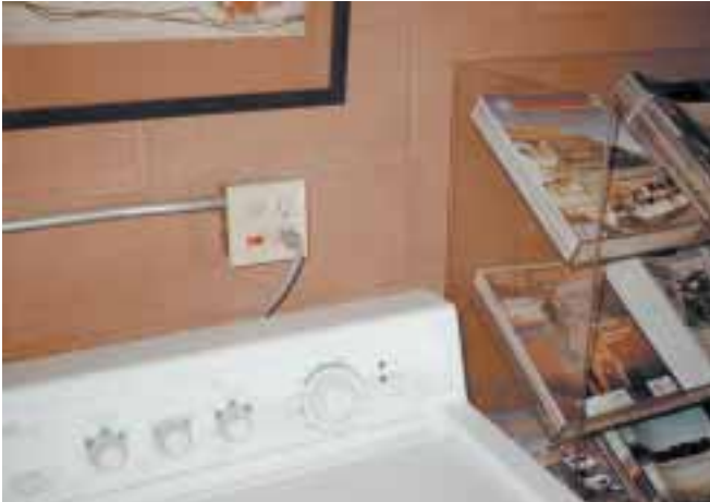
This switched outlet conveniently manages phantom loads.
