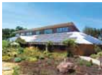
42 kW line tie powers organic wine production facility at Felzer Vineyards, provided by Real Goods.
