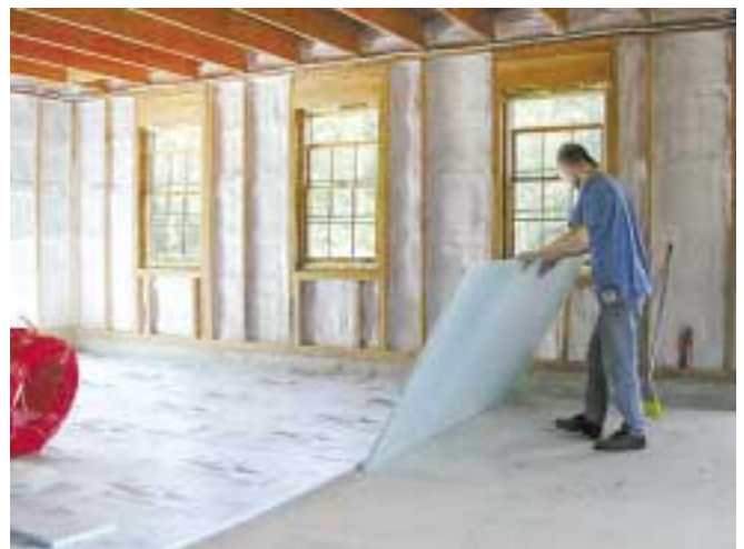
Laying 1 inch polystyrene insulation board over the old floor insulates the heated slab from the earth.
