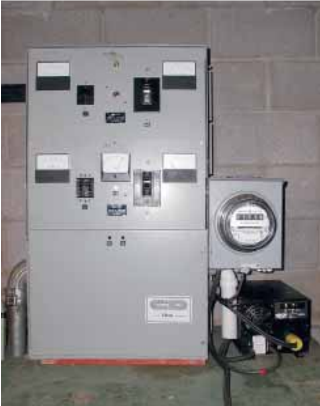
The DC power panel with breakers and meters, kilowatt-hour meter, and Tripp Lite 2,400 watt inverter.
