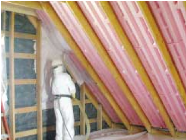
Corbond spray-on foam insulation has an R-value of about 7.3 per inch.
