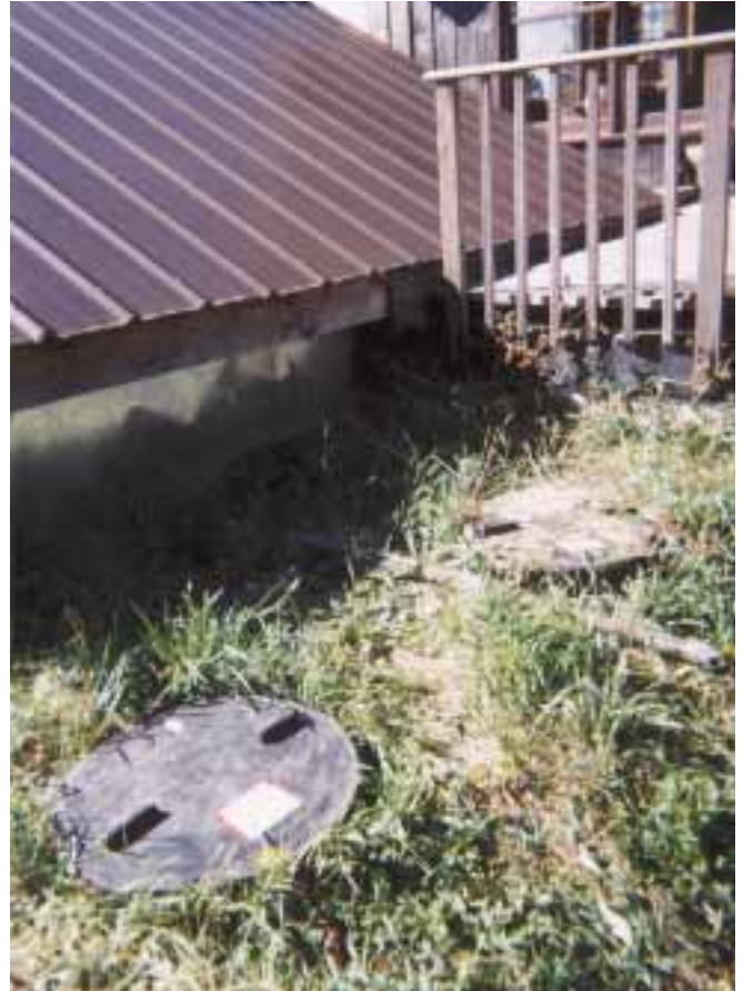
The buried tanks are unobtrusive, with only the access covers showing.
