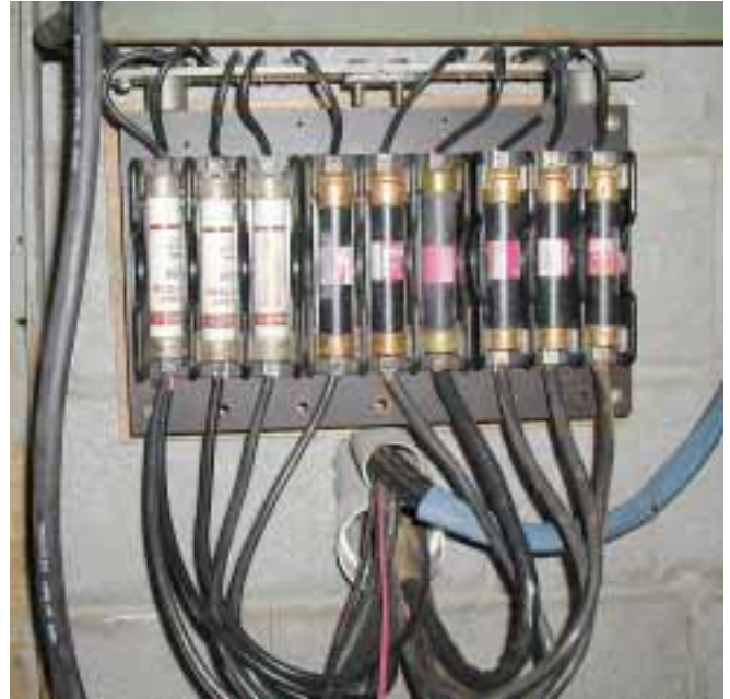
Individual 30 amp fuses for each series string of lead-calcium batteries.
