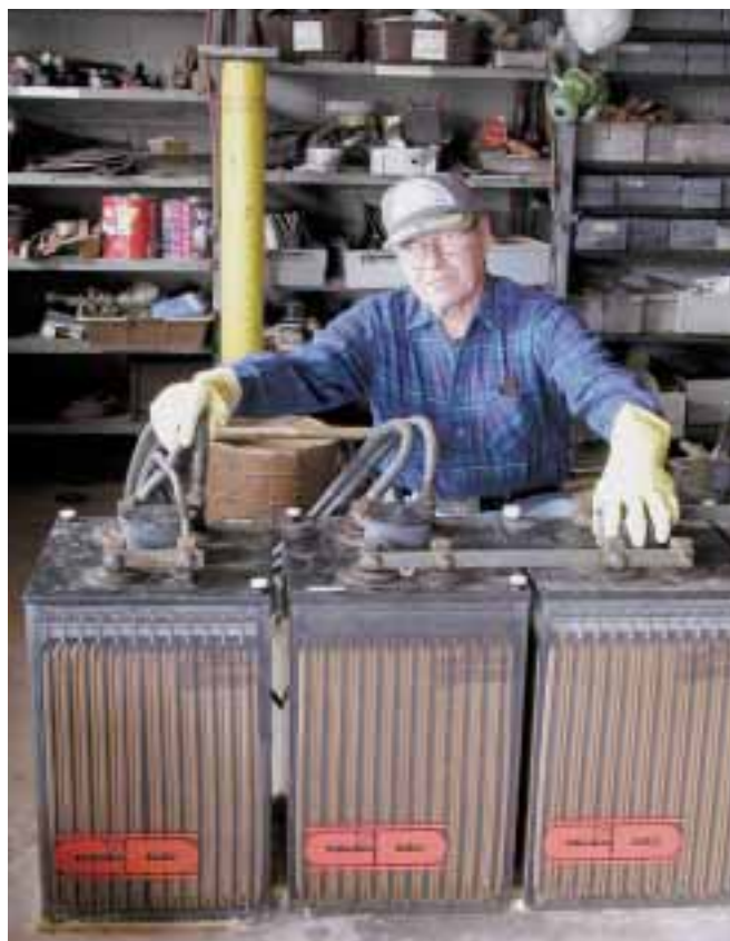
Twelve huge 2,016 AH batteries make up a single series string at 24 volts DC.
