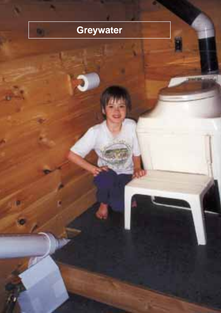
Tremayne shows off the Sun-Mar toilet, which is raised above a custom-built, 64 cubic foot composting bin.
