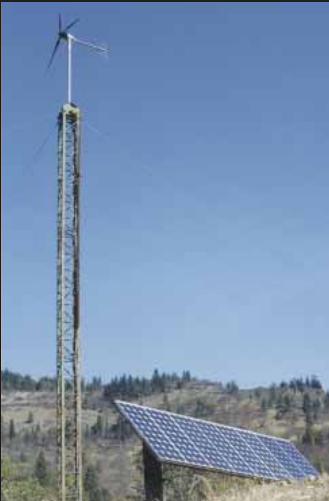
A Whisper H900 wind genny with 600 watts of PV meet the family's power needs.
