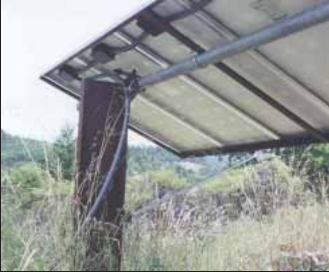
The underside of the PV rack showing its homemade mounts.
