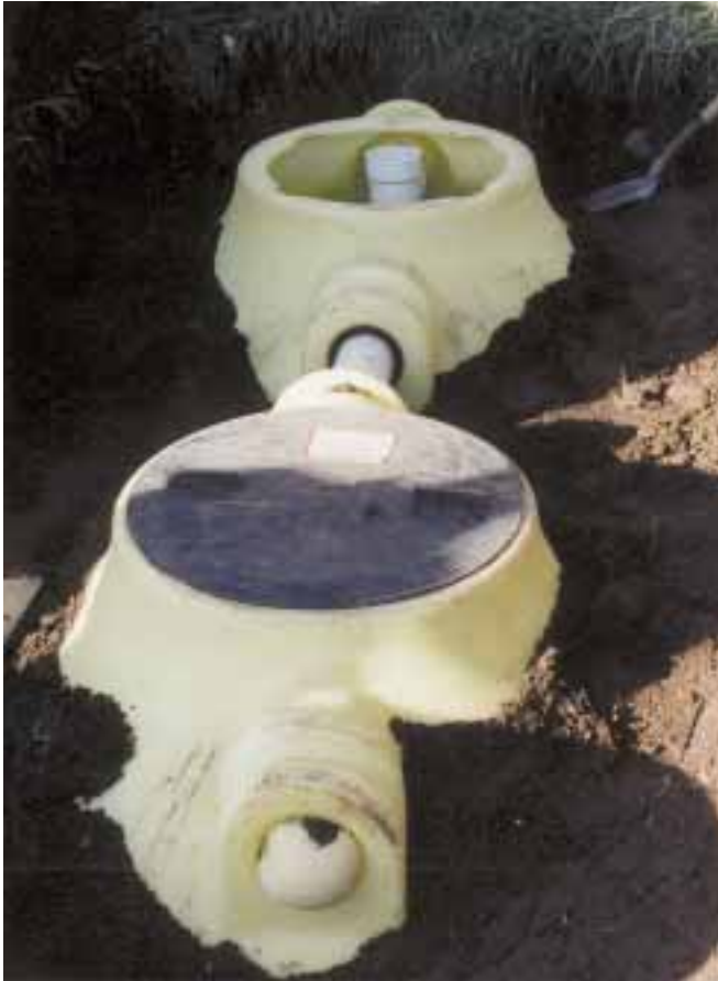
Two Norwesco plastic sphere tanks help settle and filter greywater before irrigation.
