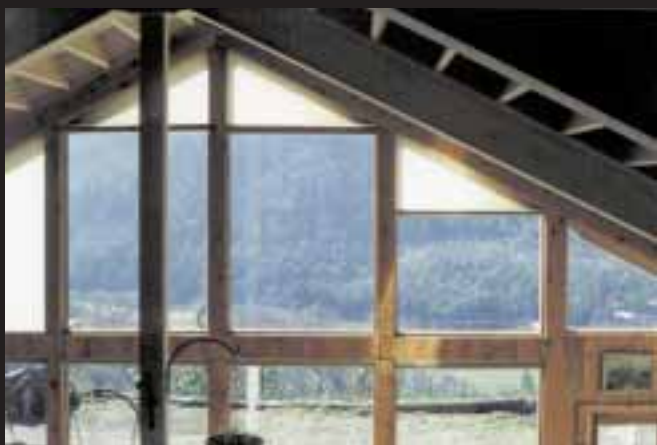
The loft's view—the passive solar design includes a window-to-floor ratio of about one to eight.
