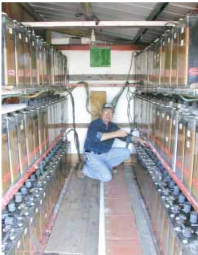
Peter's packed battery room holds over 5,000 amp-hours of lead calcium-batteries at 24 volts DC.
