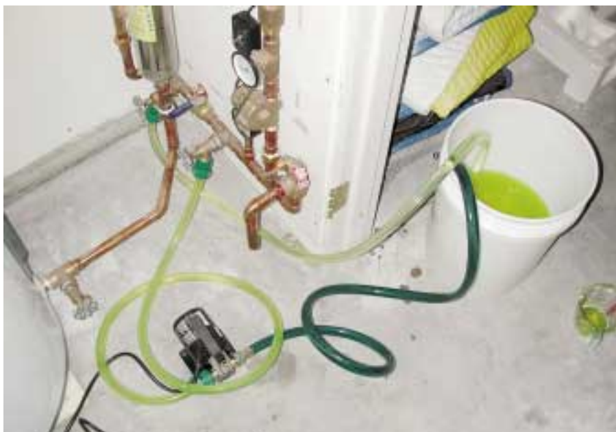
That's not Gatorade! Filling and pressurizing the solar collector loop with the propylene glycol solution.
