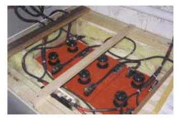
Three of the twelve Rolls batteries. The #4 (21 mm<sup>2</sup>) wiring shown is from the C60 controllers.
