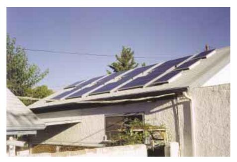
From three panels to twenty-five—the system keeps growing, and growing, and growing! The sixteen KY120, seven KY80 and two SP75 PV panels.
