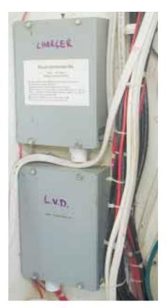
The voltage sensors and controls for the low voltage disconnect and AC battery charger. press, and the winnowing machine, are routed through 75, 75, 45, and 30 amp DC-rated breakers, respectively, in the load center.
