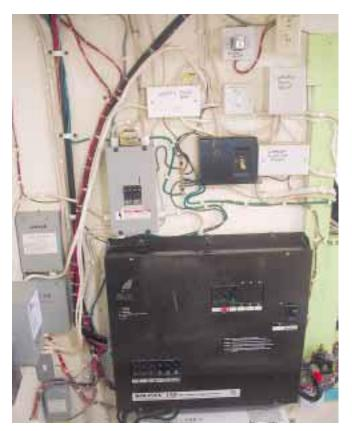
The power wall including the SolPan 110 DC load center, which contains a Heliotrope CC-120 charge controller.
