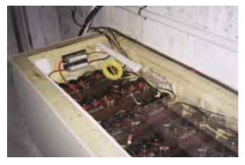
Eighteen Trojan T-105s make up this battery bank. The battery system is insulated, fused, and vented.
