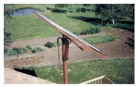
The PVs' top-of-pole mount eliminated the potentially dangerous roof mount.
