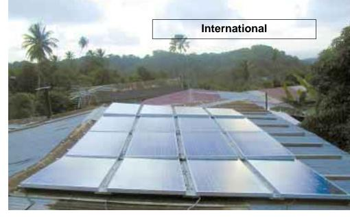
Sixteen, 120 watt AstroPower modules provide power directly to DC-driven, chocolate making machines.
