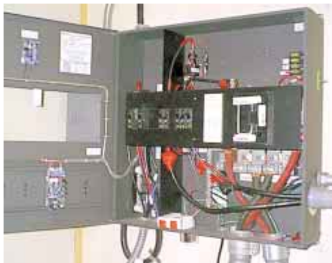
Inside the Ananda Power Center you can see the main pullout DC disconnect, DC breakers, and the backs of the TriMetric and Smart Charger.
