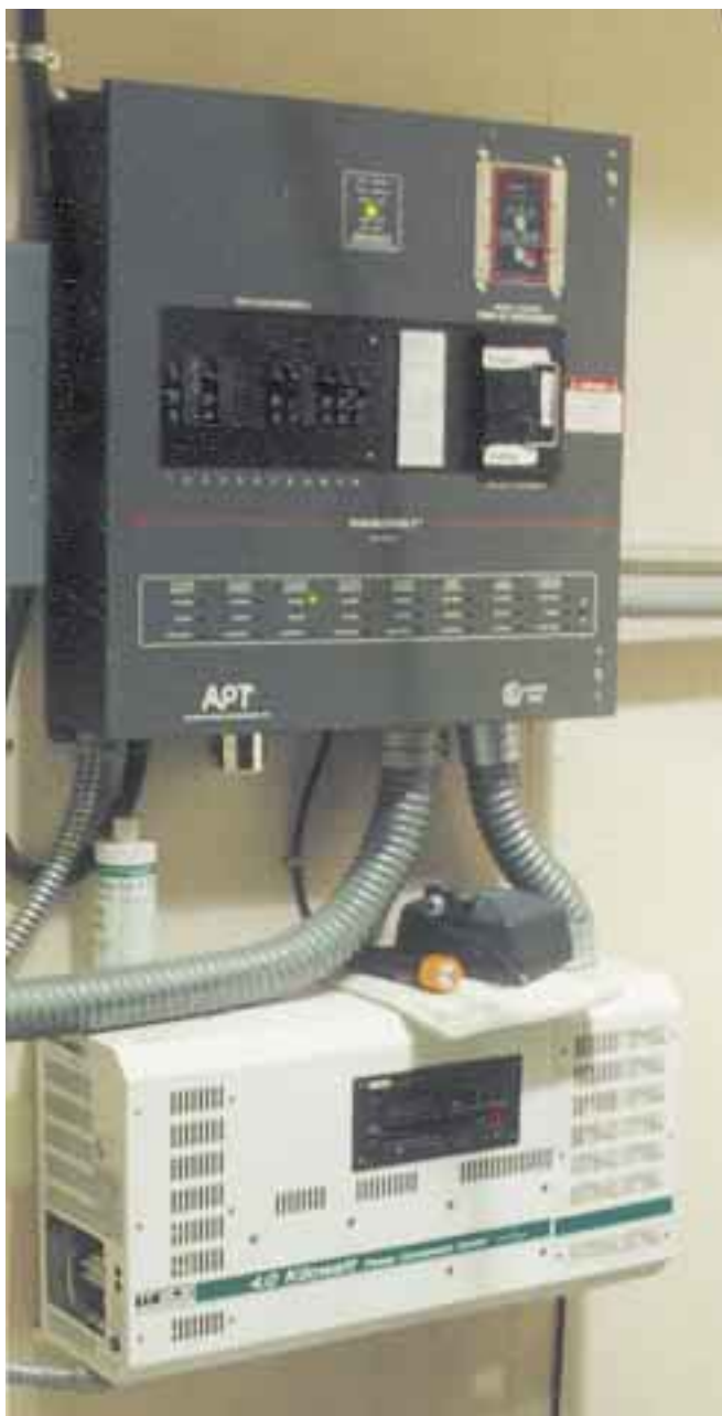
The Ananda Power Center and Trace SW4024 came prewired and were bought used.
