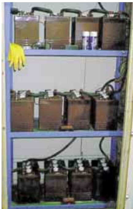
Twelve of the sixteen Trojan T-105 lead-acid batteries that provide 880 amp-hours of storage.
