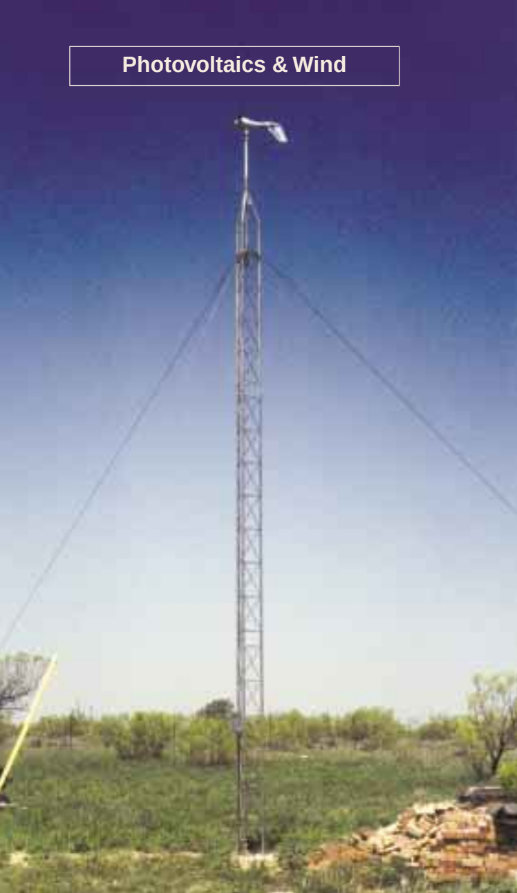
The Southwest Windpower Air 403 on a 30 foot tall Rohn 25G tower.
