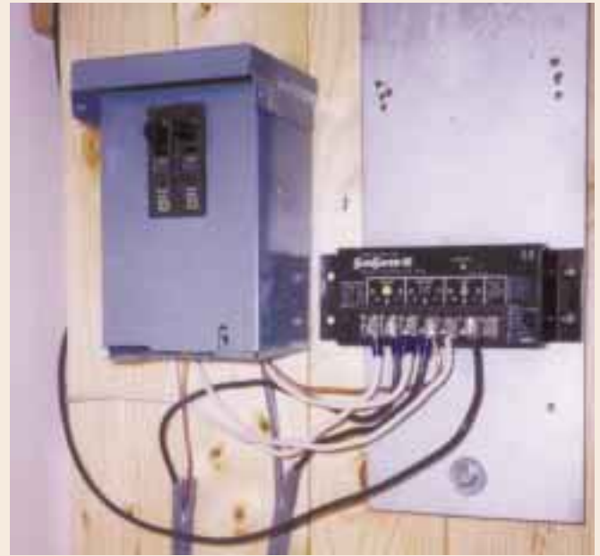
Breakers and the Morningstar SunSaver-10 charge controller for the 12 volt system.
