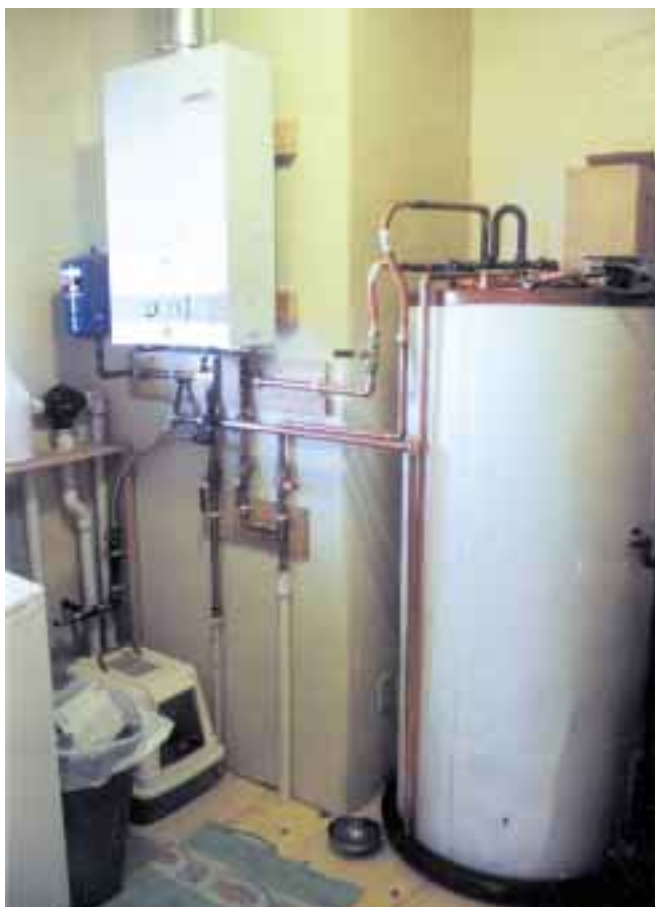
An Aquastar BS on-demand water heater (upper left) backs up the solar hot water system.
