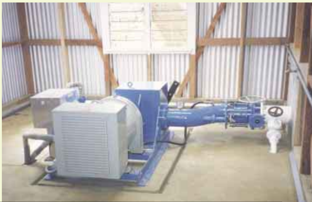
A typical Canyon Pelton (75 KW ) in a remote area of Papua New Guinea.
