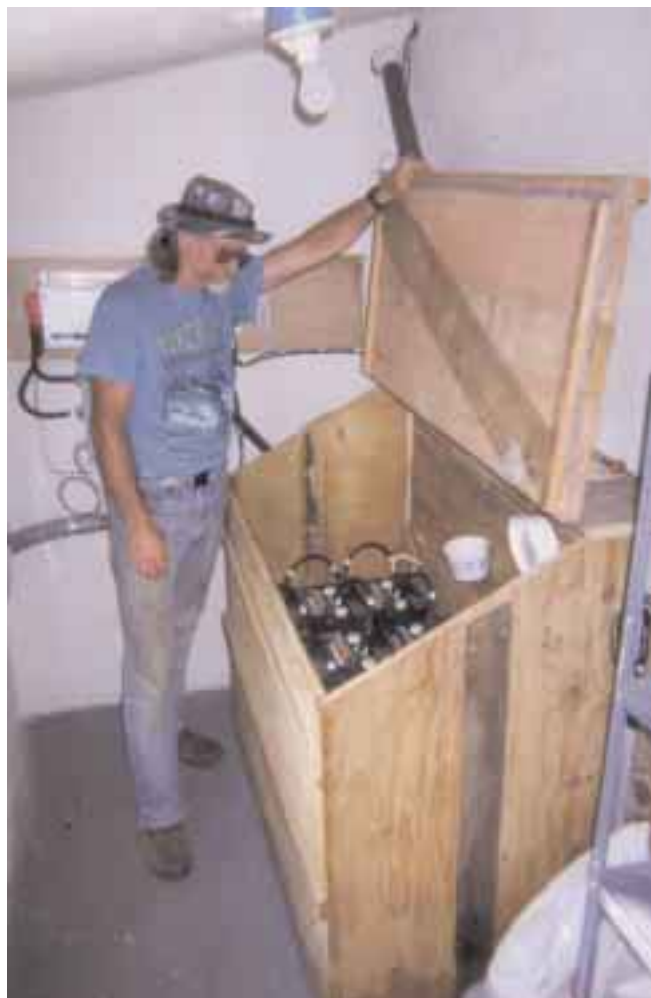
The vented battery box is built onto two small pallets to keep the batteries off the floor. Twelve Interstate 6 volt, 350 AH batteries provide 1,050 amp-hours at 24 volts.
