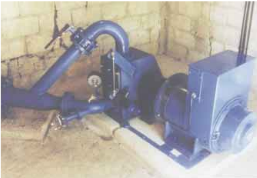
A 15 KW Pelton turbine operating in Costa Rica.
